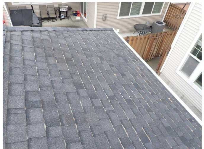
#42 Minor moss build up on roof surface, moss appears to have been treated.
