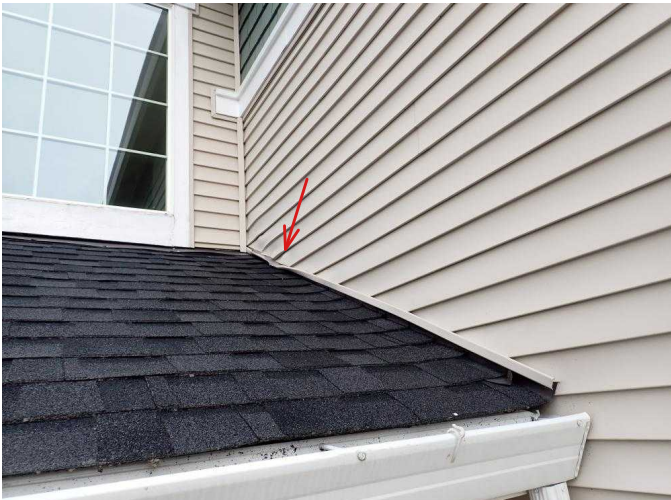
#25 Lower vinyl J-track on E side of front porch door is bent.
