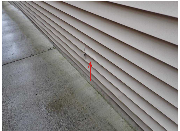
#16 Minor buckling in lower E siding.
