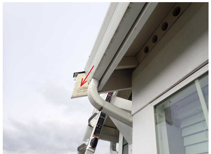
#30 Paint peeling in lower fascia tails.
