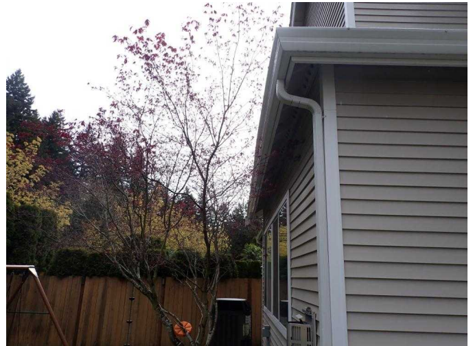
#14 Tree in contact with lower N roof needs to be trimmed back.
