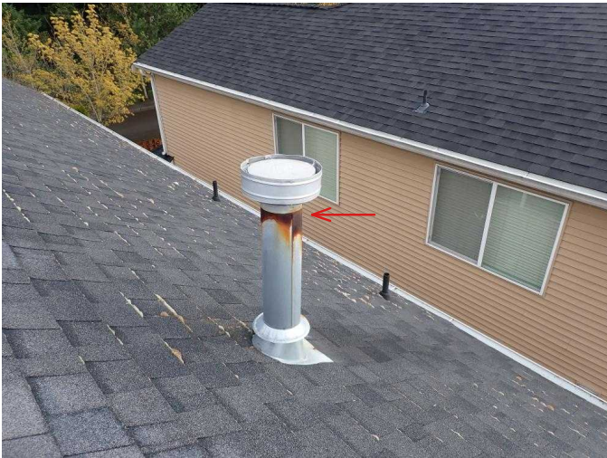
#31 Exterior section of furnace flue starting to rust and will need to be replaced in next 5 years.
