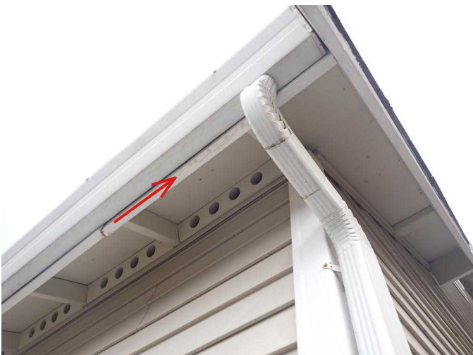
#23 Water behind E end of attached garage gutter indicates roof water is getting between gutter and garage fascia board.
