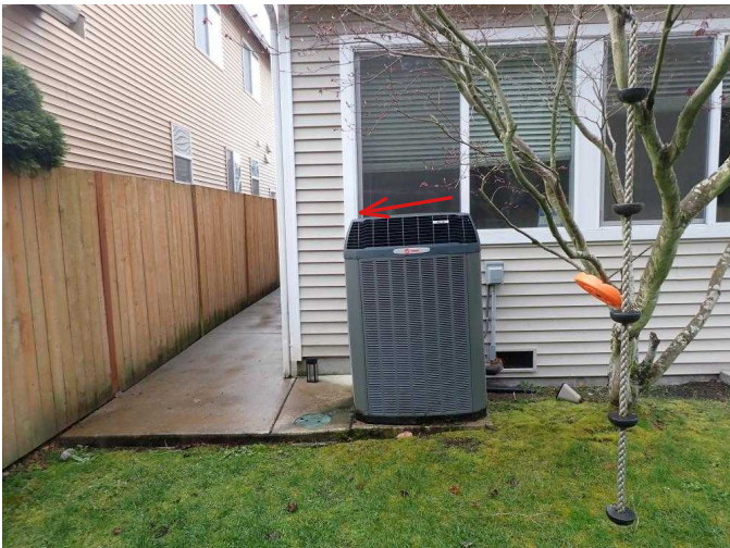
#15 Support pad for heat pump exterior unit is not level, exterior unit needs to be level to reduce stress load on
