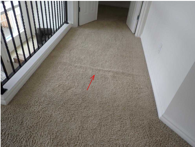
#79 Minor buckling in second floor hallway carpet. (added)
