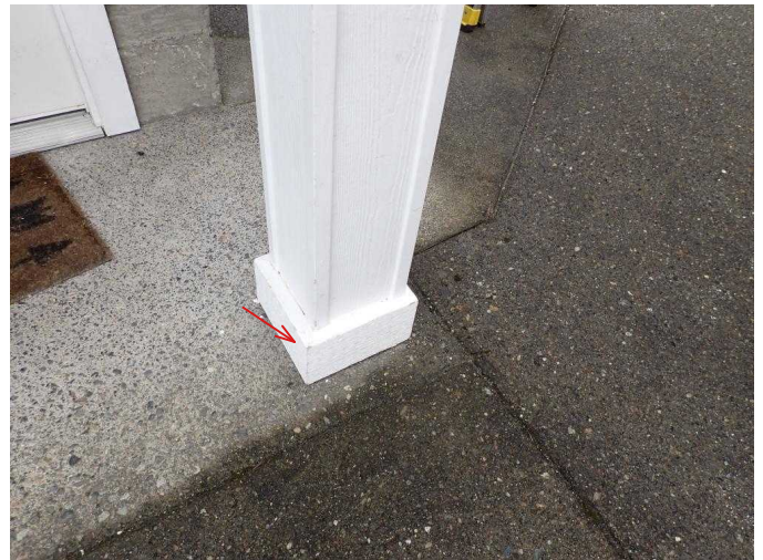
#40 Minor paint peeling in wood trim work.
