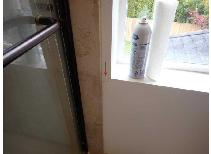
#92 Cosmetic crack in wall material next to master shower.
