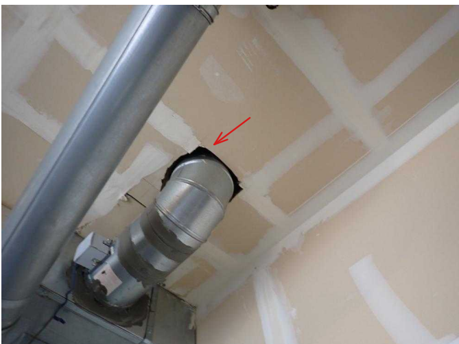
#59 All open holes and gaps in ceiling need to be sealed against fire intrusion if a vehicle is to be parked in the garage.
