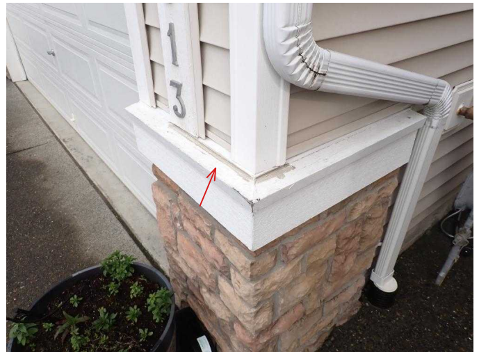
#22 Minor paint peeling in wood trim system.
