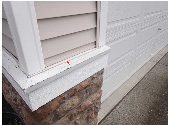
#2 Minor paint peeling in sections of wood trim work.
