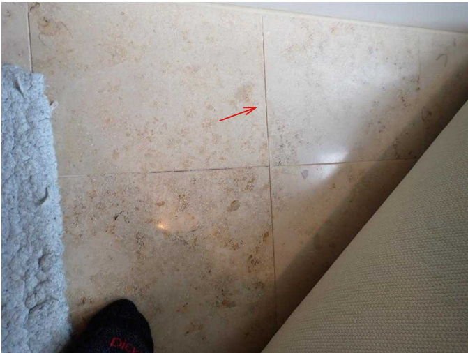
#85 Sections of grout missing in front of shower in master bathroom.
