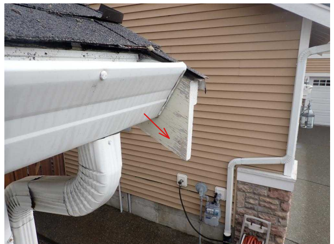
#24 Minor paint peeling in lower fascia tails.
