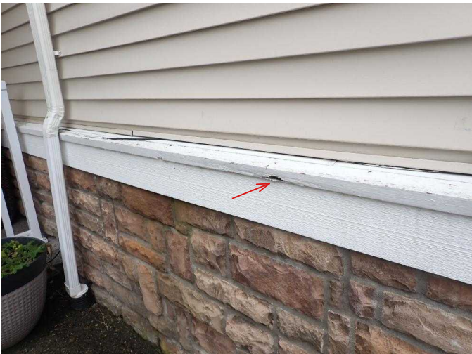
#3 Minor rot occurring in W wood trim on attached garage exterior.
