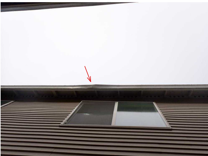
#17 Moderate dent in E gutter system.
