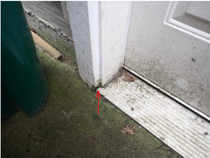
#19 Rot occurring in attached garage door trim where in contact with cement.
