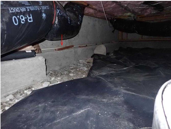
#67 All construction debris in crawl space should be removed.
