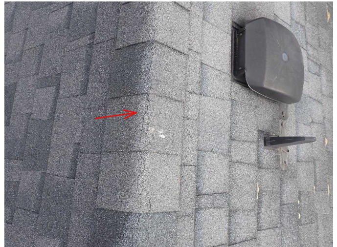
#32 Minor cracking in ridge cap material.
