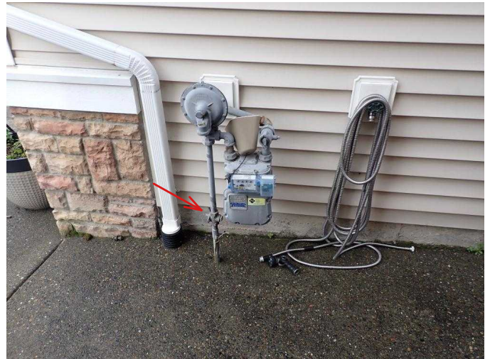
#20 Gas main shut off valve at meter located on the E side of the house.
