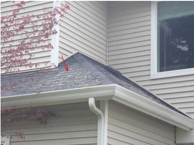
#13 Moderate moss build up on roof, moss appears to have been treated.
