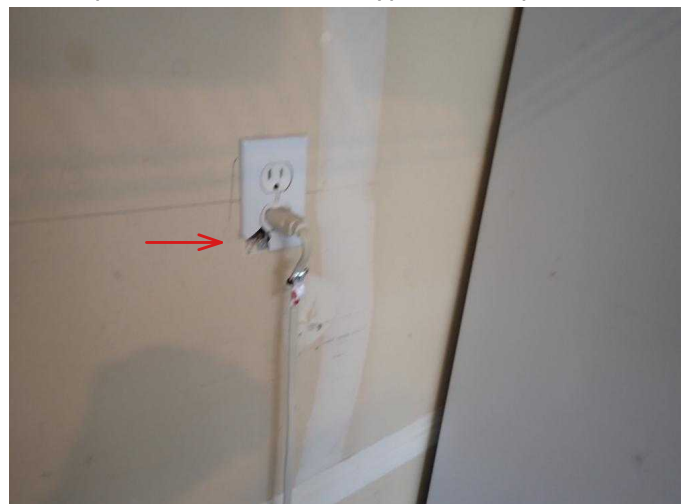
#54 Outlet cover plate broken in garage, should be replaced.
