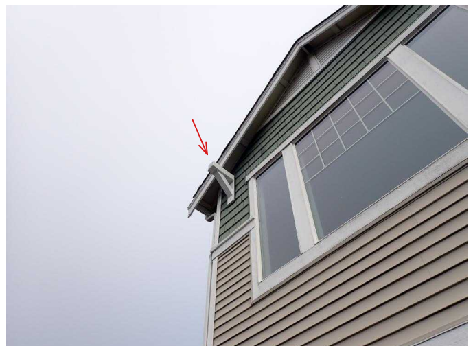
#6 Ends of knee brace trim work, protruding into weather from soffit areas.
