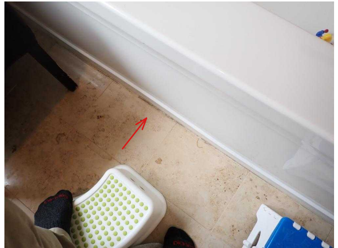
#86 Caulking needs to be redone at floor/tub junction in master bathroom.
