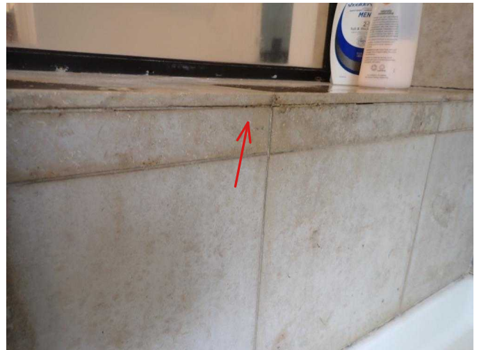
#88 Small sections in grout missing in front edge of shower seat in master bathroom.
