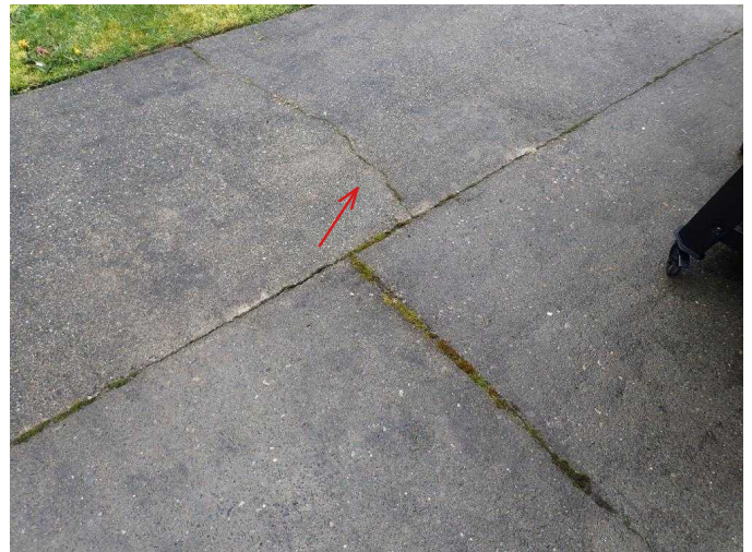
#10 Minor cracks in N patio surface are present with minor settling.
