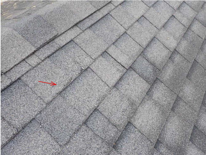
#43 Roof is moderately worn with small sections of fiberglass mesh exposed.
