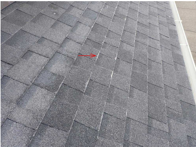
#27 Roof is moderately worn with small sections of fiberglass mesh exposed.
