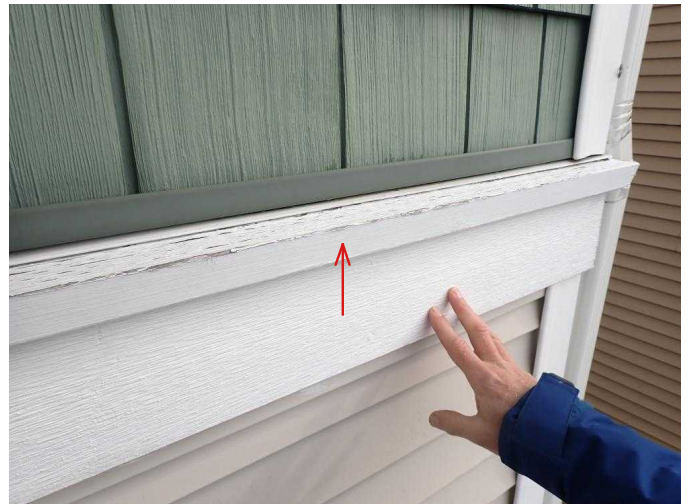
#28 Minor paint peeling in wood trim system.
