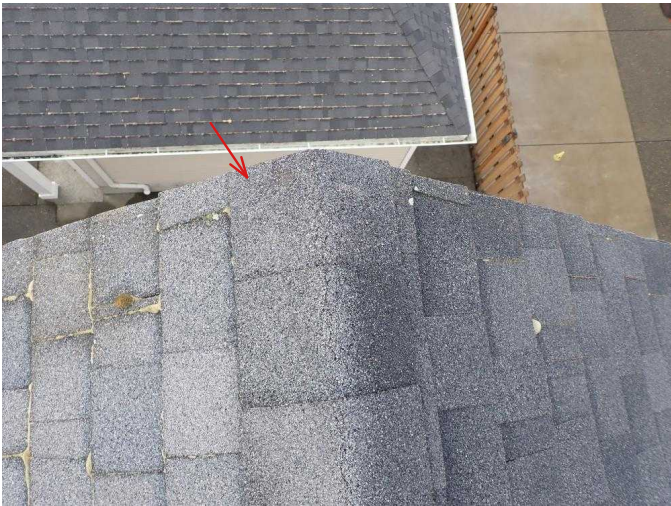
#37 Moderate wear in roof system.
