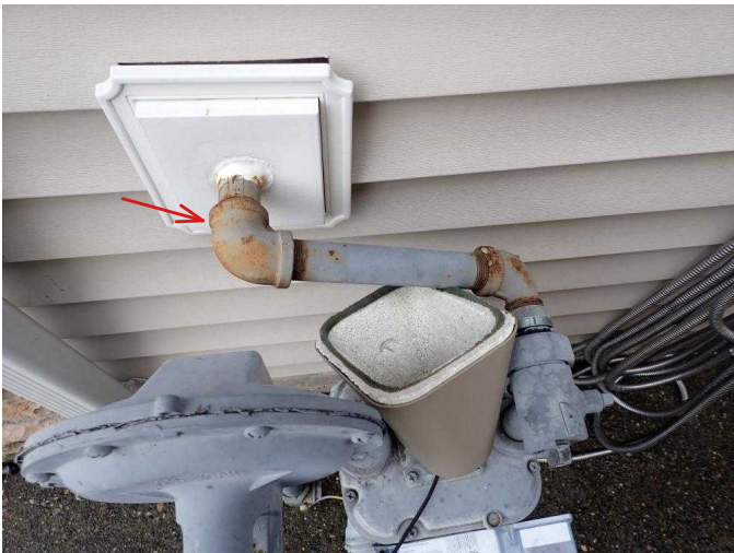
#21 Exterior sections of gas lines are rusty.
