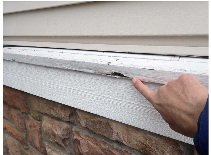
#4 Minor rot occurring in W wood trim on attached garage exterior.
