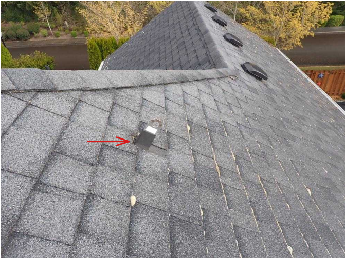
#33 NE safety anchor is missing weather cover on roof.
