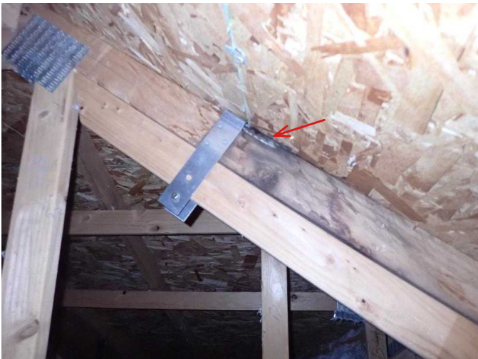
#63 Minor rot and staining in 2X4 truss system and sheathing material at NE safety anchor, visible in attic.
