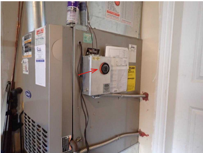
#57 Timer for whole house fan located on furnace.
