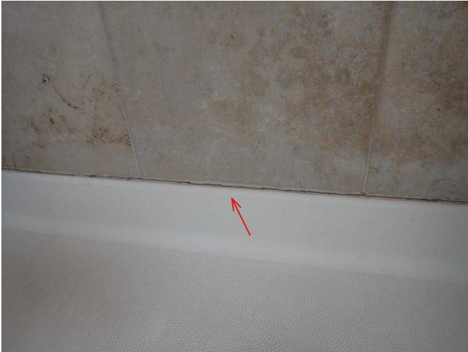
#91 Caulking needs to be redone at pan/surround junction in master bathroom shower.
