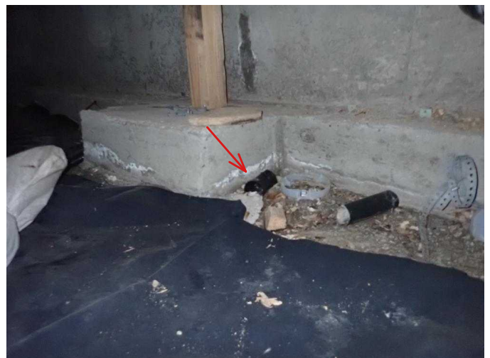
#66 All construction debris in crawl space should be removed.
