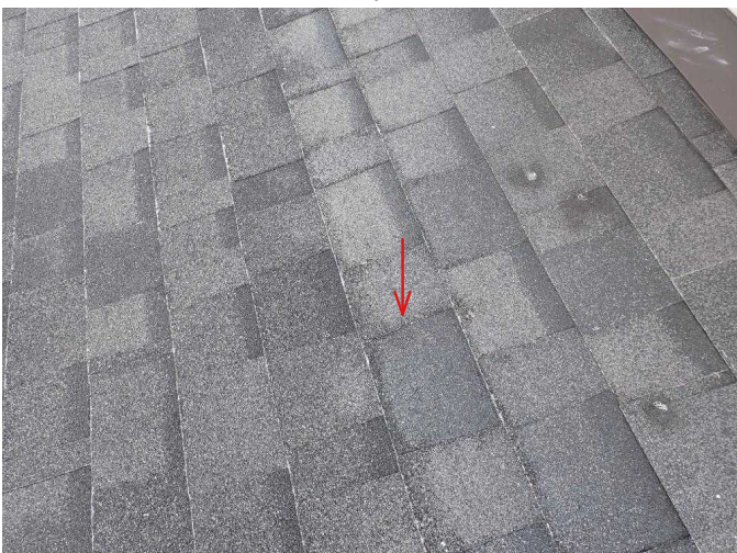
#29 Roof is moderately worn with small sections of fiberglass mesh exposed.
