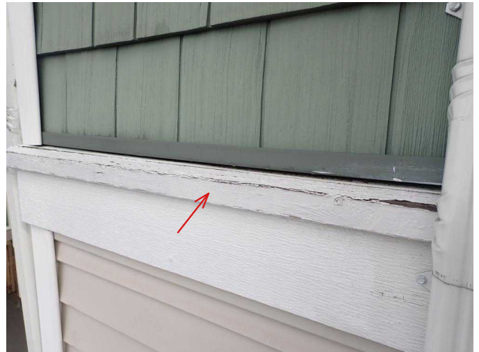
#26 Minor paint peeling in wood trim system.
