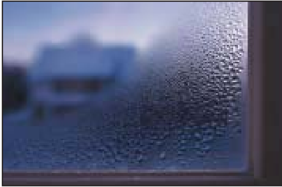
Condensation on the inside of a windowpane.
